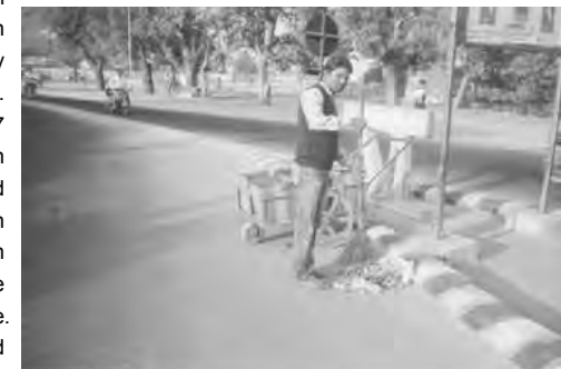
Use of containerized handcart and long handled broom for street sweeping
