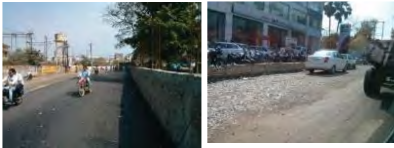
Figure 44: Improvement initiative taken up by the city (Road Widening)
