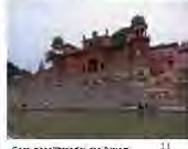
Grant installed by the Project
