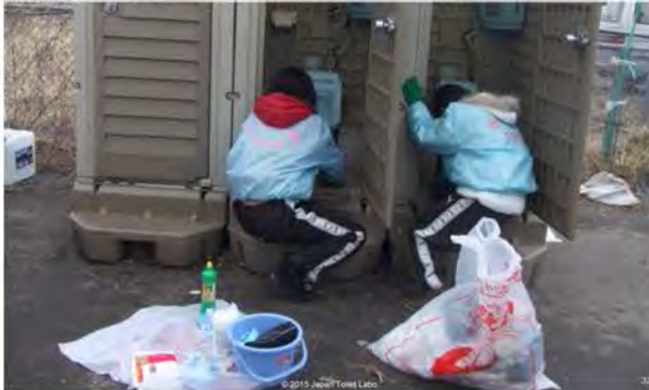
A project team for improvement school toilets (Miyagi, Japan 2011)
