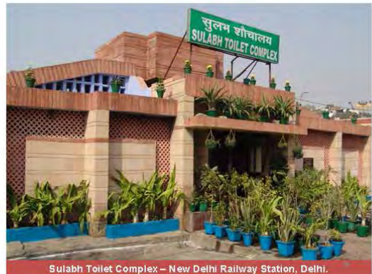
Sulabh Toilet Complex – New Delhi Railway Station, Delhi.
