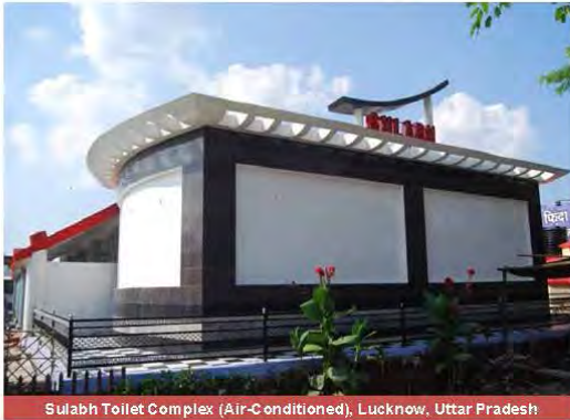
Sulabh Toilet Complex (Air-Conditioned), Lucknow, Uttar Pradesh
