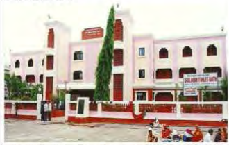
Largest Sulabh Toilet Complex in the world at Shirdi (Nasik), Maharashtra, India
