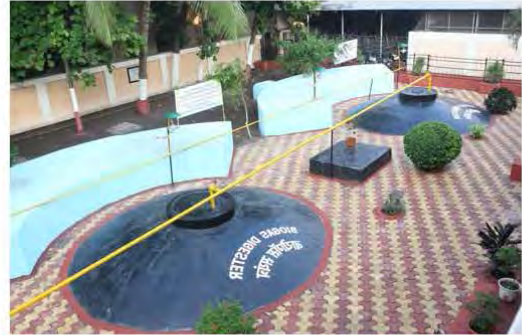
Biogas generation at Sulabh Toilet Complex, Shirdi, Nasik, Maharashtra
