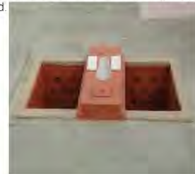
Sulabh pour-flush toilet for least space with the toilet on top of the pits
