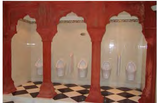
Urinals inside Sulabh Toilet Complex, The Taj Mahal, Agra. This was declared second best in the world. (Hindustan Times, 12th July 2006)
