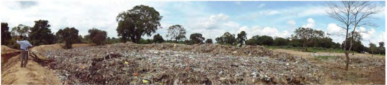
Active filling area
