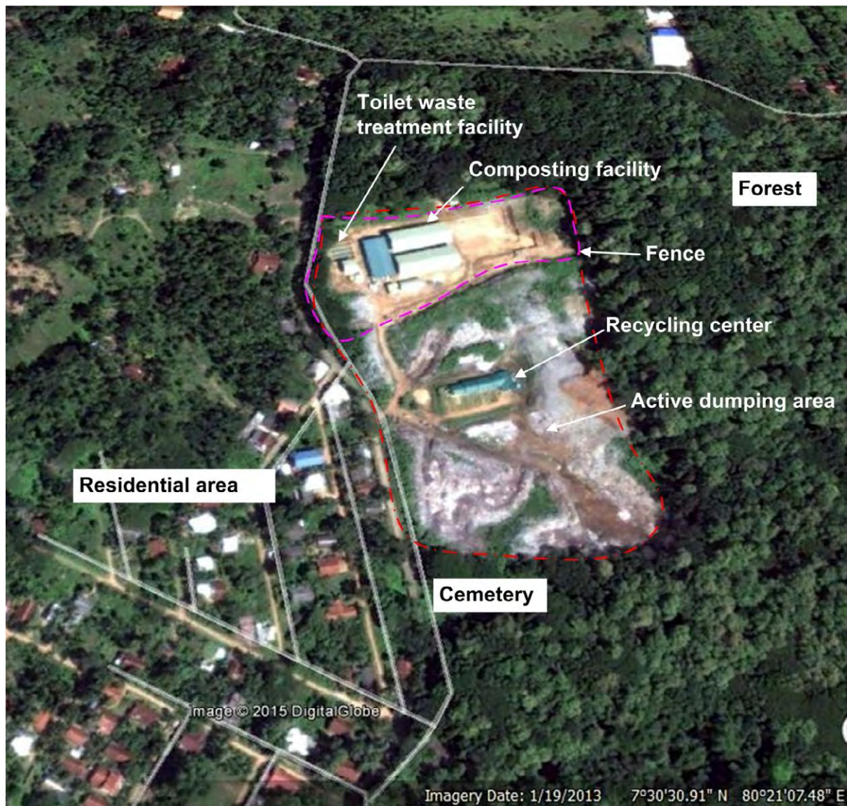
Figure 4-2 Sundarapola dumpsite and environment within 500 m radius from center
