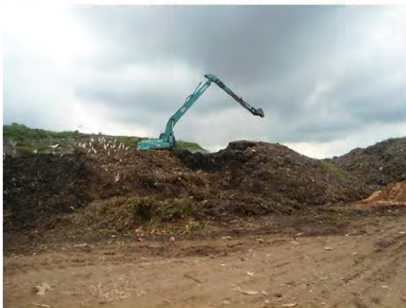
Excavator (long arm)
