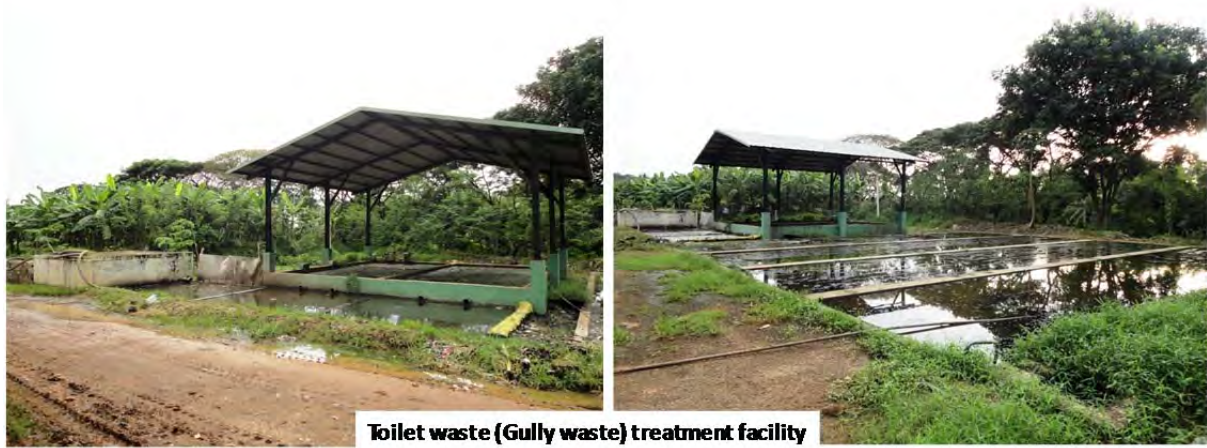
Figure 4-7 Toilet waste treatment facility at Sundarapola dumpsite
