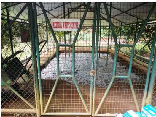
Medical waste disposal facility
