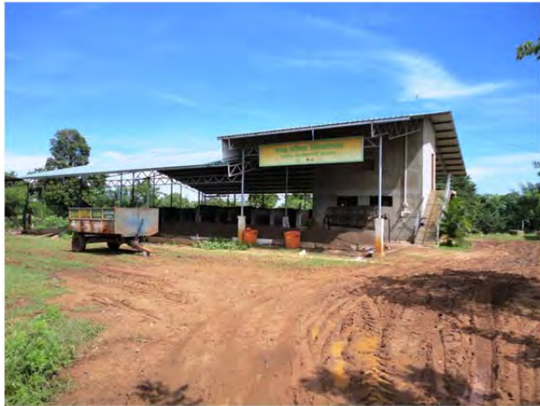
Composting facility- Kataragama Ps
