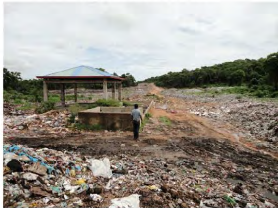
Toilet waste treatment facility
