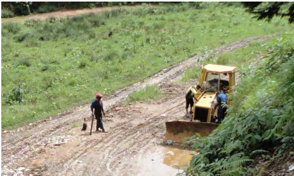
Figure 4-4 Landfilling machineries at Moonplains dumpsite
