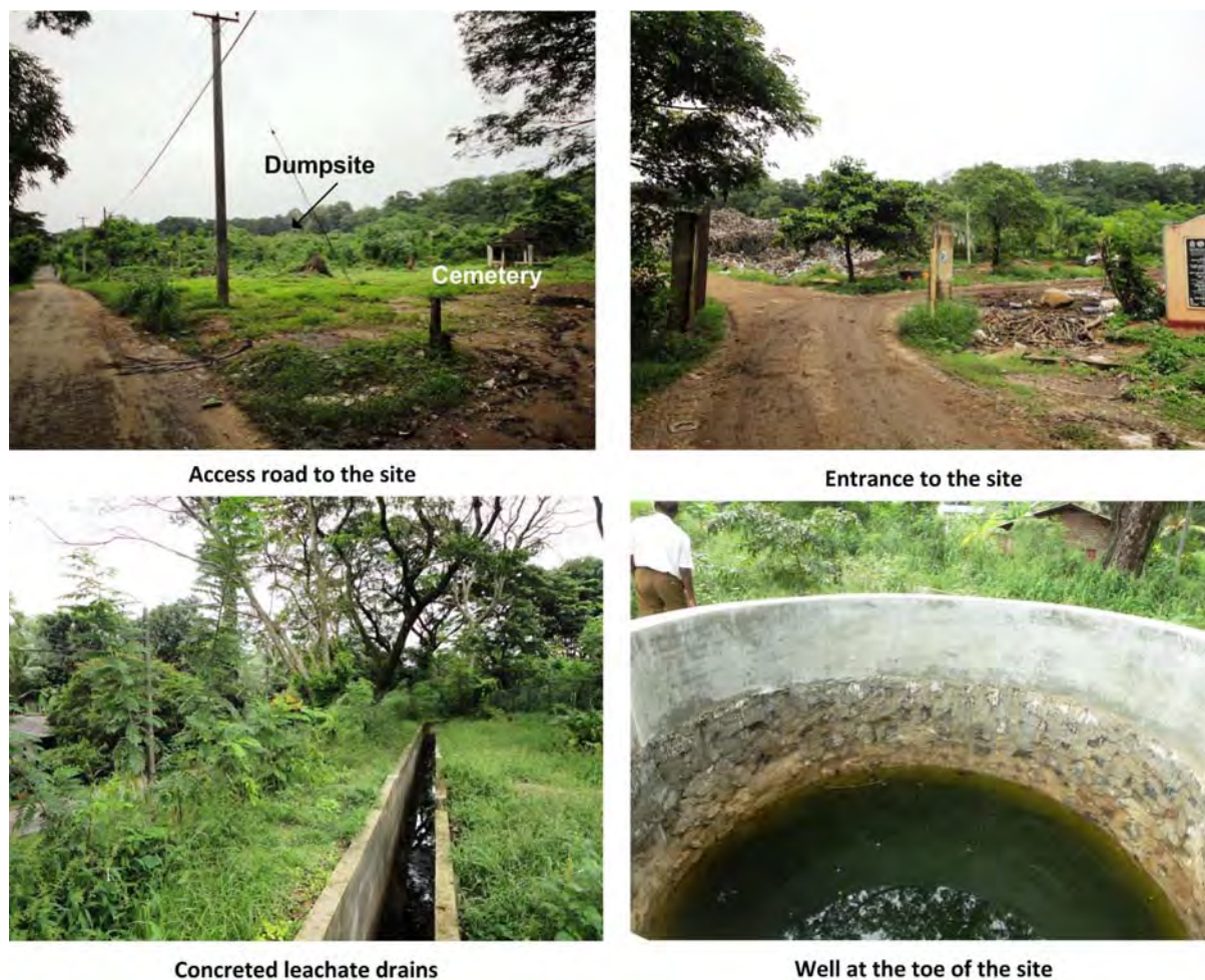
Figure 4-3 Access road and basic site infrastructure facilities at Sundarapola dumpsite
