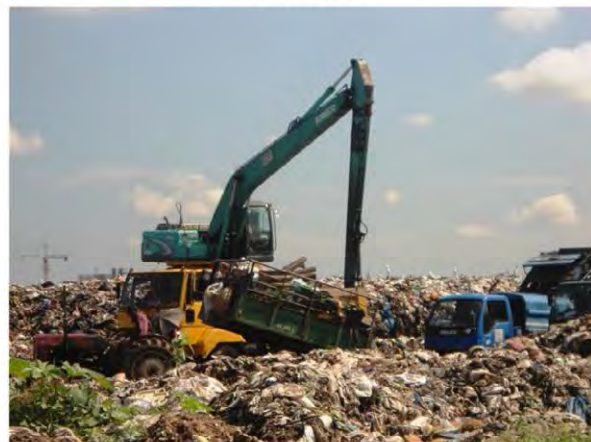
Excavator (long arm)
