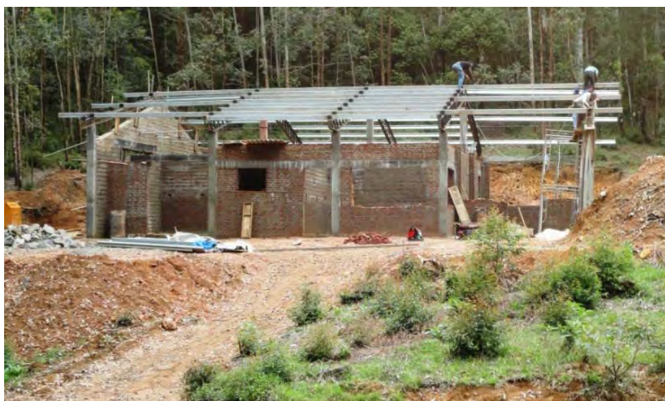
Figure 4-6 Plastic recycling center under construction
