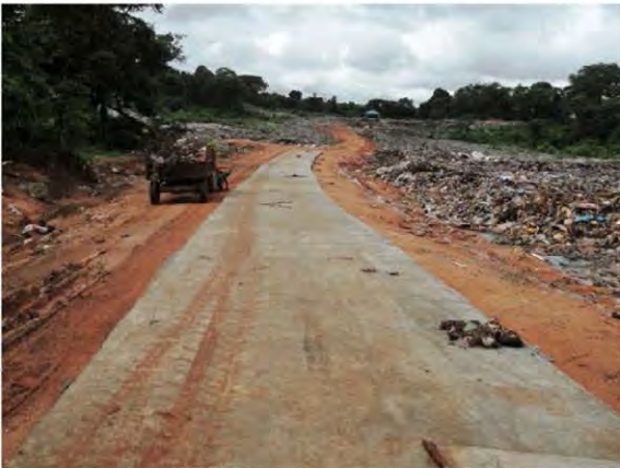
Newly paved access road near the dump
