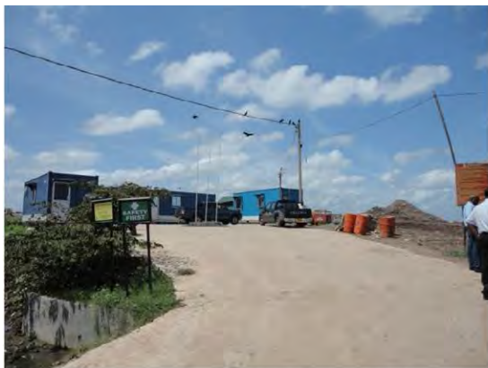
Site infrastructure buildings
