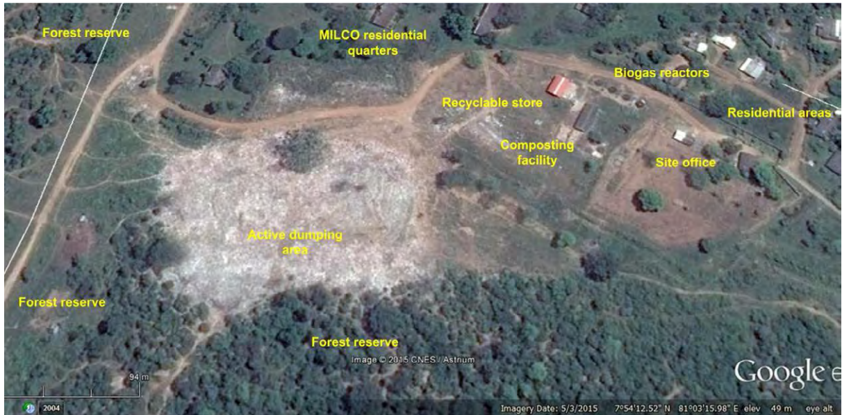
Figure 5-2 Environment around the Thamankaduwa MSW disposal site
