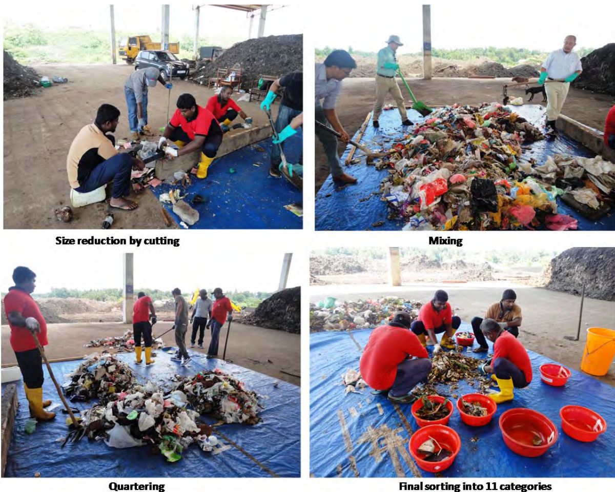
Figure 2-2 Particle size reduction, mixing and preparation of working sample by coning & quartering technique
