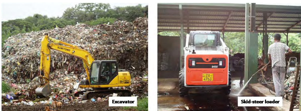
Figure 4-4 Landfilling machineries at Sundarapola dumpsite
