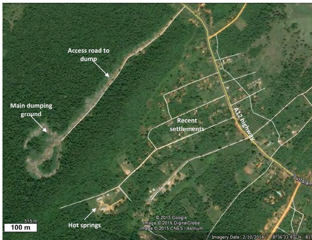
Figure 4-3 Environment around the Trincomalee UC's dumpsite
