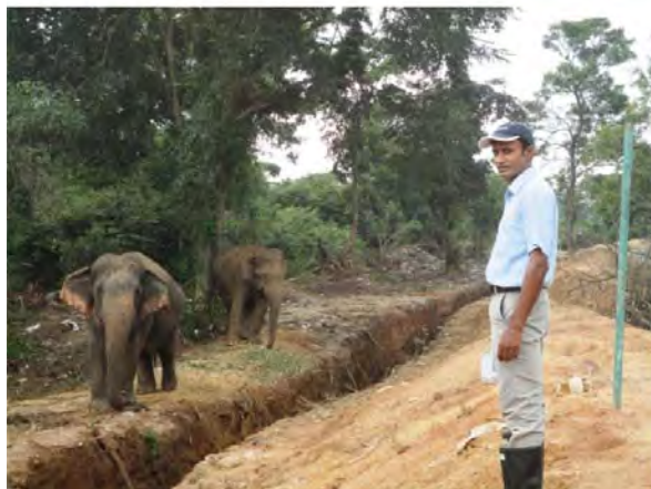
Figure 5-3 Protective measures to prevent elephants entering the site
