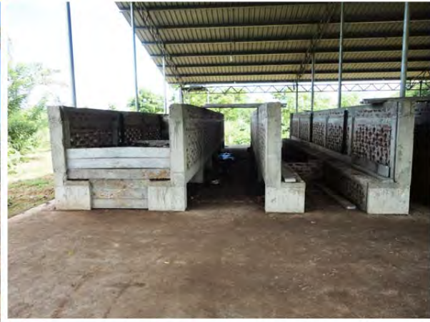
Passive aerated composting bins - Kataragama Ps
