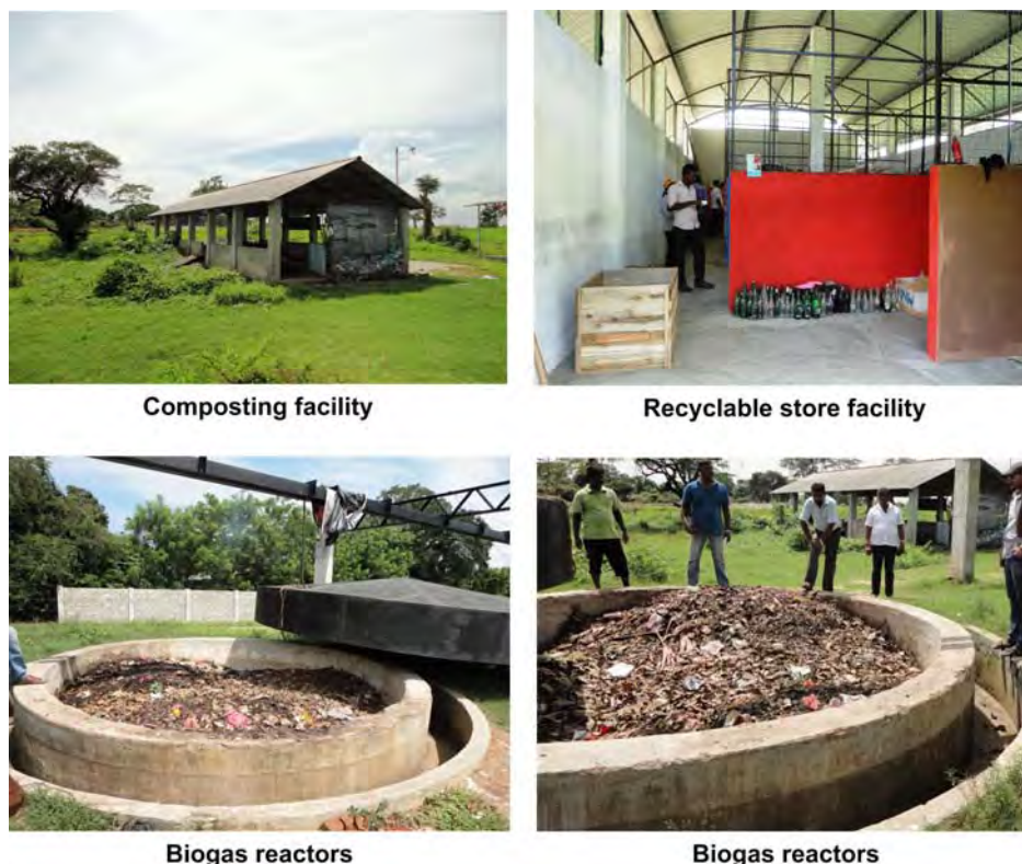
Figure 5-4 Auxiliary MSW management facilities at Thamankaduwa dump site
