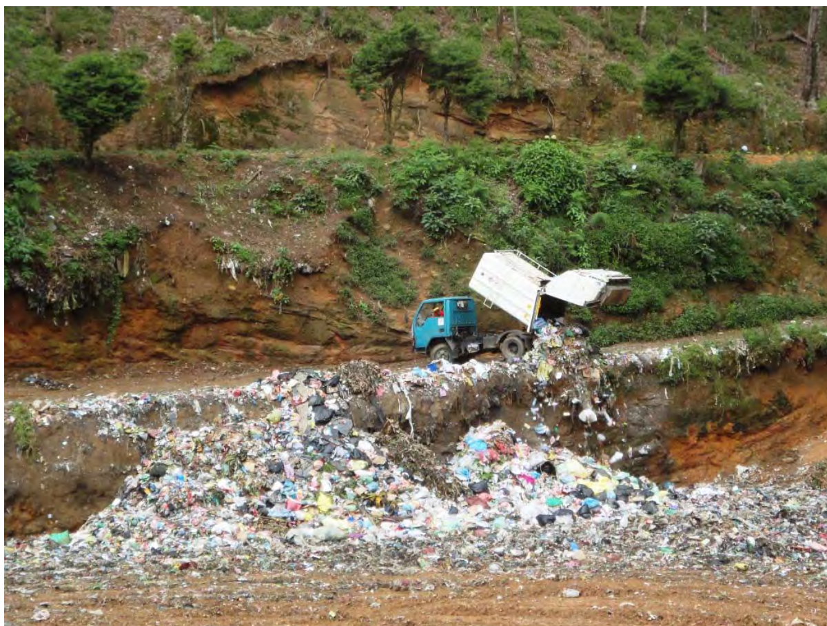
Figure 4-5 Waste unloading and dumping area of Moonplains dumpsite
