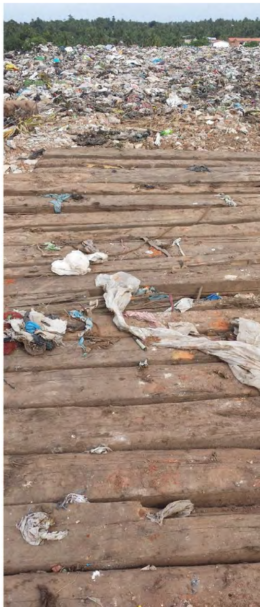
Access on the dump made by railway slippers
