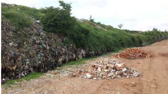
Access on the dump
