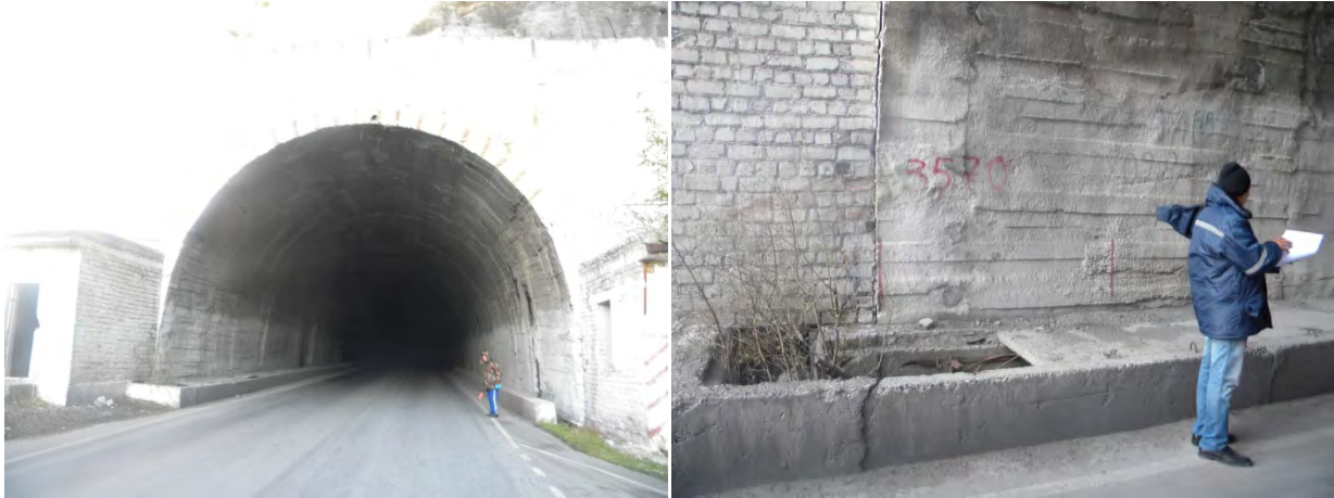
Tunnel No.2 Planned inspection (2014.10.29)
