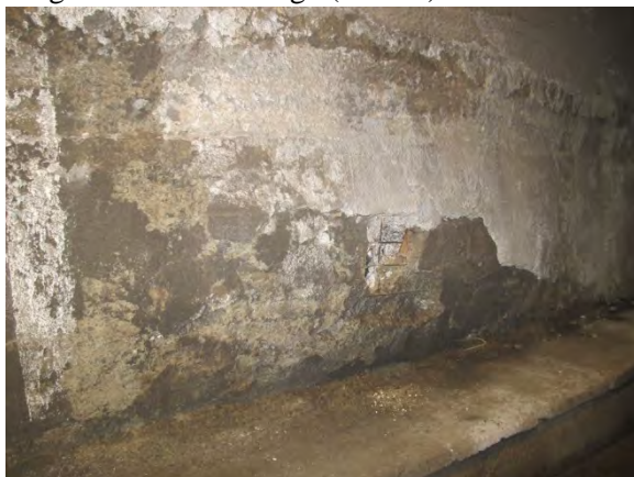
Photo 6-15 The Condition of Kolbaev Tunnel Wall Damage (2014.6)
