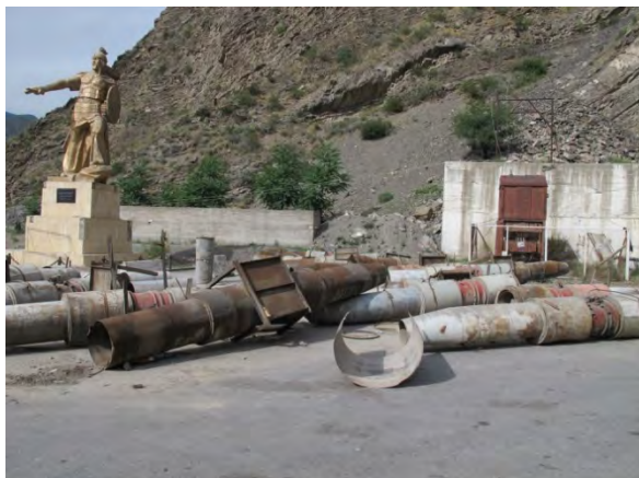
Tunnel No.3 (ventilation) (2014.6)
