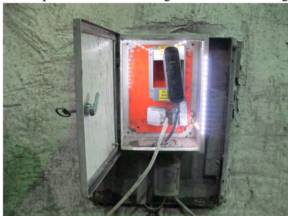
Photo 6-28 Condition of Improved Emergency Phone (2015.6)
