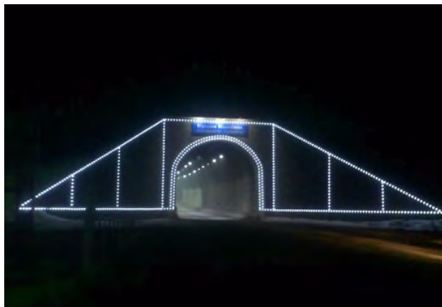
Photo 6-20 Illumination of Kolbaev Tunnel Portal (2014.6)
