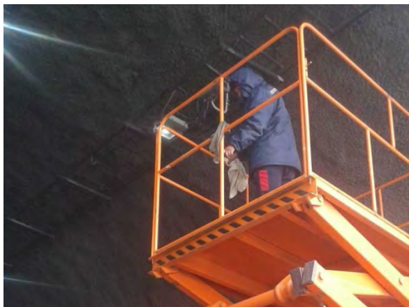
Lighting equipment cleaning
