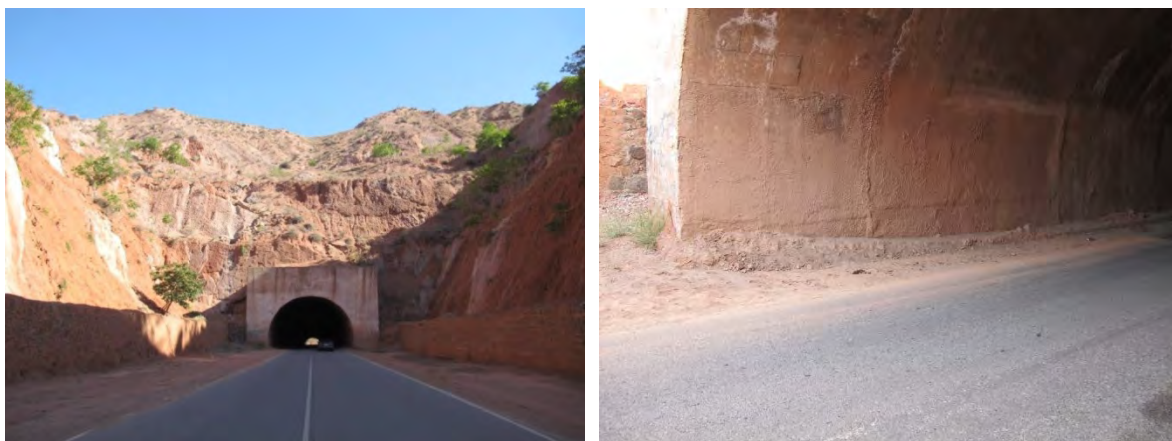
Photo 6-17 The Situation on Osh Side Portal of Tashkomur Tunnel Osh (2013.8)
