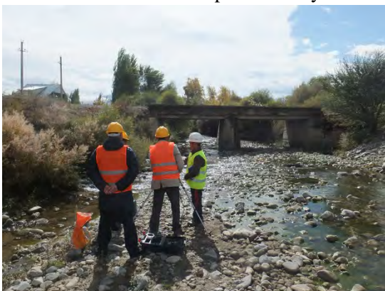
Photo 5-8 Training on Planned Inspection B at Site
