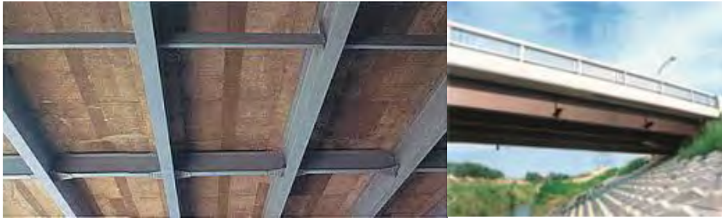
Figure 12.6.8 Construction Examples of an H-shaped Steel Bridge
