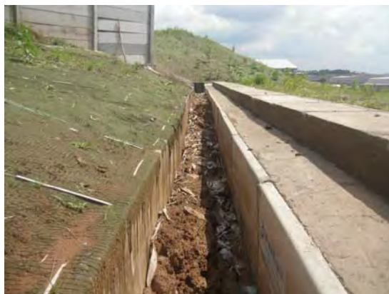
Photo 10 The soil outflow situation (Other company sheet)
