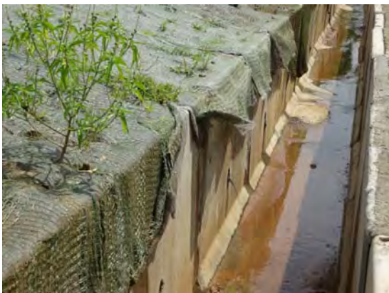
Photo 9 The soil outflow situation (SP-60)
