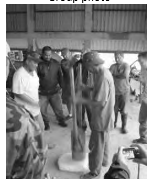
Demonstration of how to compact the "Do-Nou" bags
