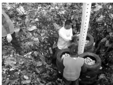
Training to install gas venting pipes
