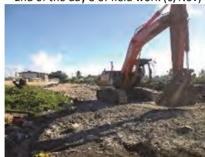
Constructing the approach road with coral sand (11/Nov)
