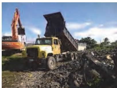
Transporting the waste by the dump truck and compaction by the excavator
