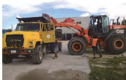
Loading the waste to the truck using the wheel loader
