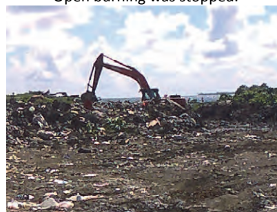
Compaction by using the excavator
