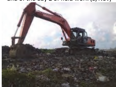
Compaction of the waste by the excavator
