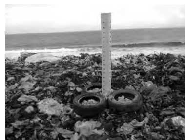
The gas venting pipe which installed
