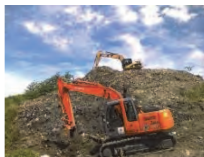
Formation of the approach road and dumping stage
