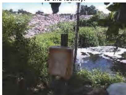
The joint box for wiring of the leachate recirculation pump
