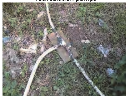
The PWMS installed cocks for the leachate recirculation
