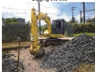
Installation of the gravel bed
