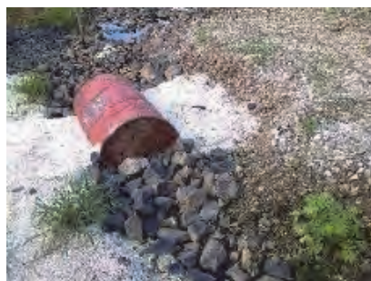
A filter process by using empty drum has been added to the facility.
