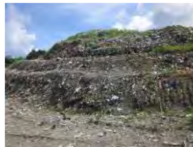
waste shaped with terraced slope
