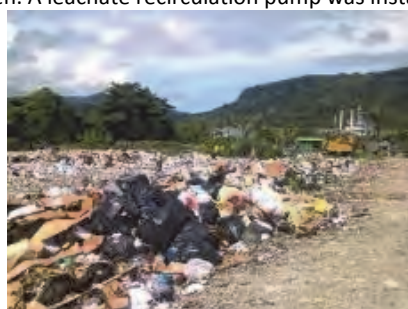
No compaction since the compactor is under repaired for two months. Maintenance of the equipment is one of the big issues on the operation.
