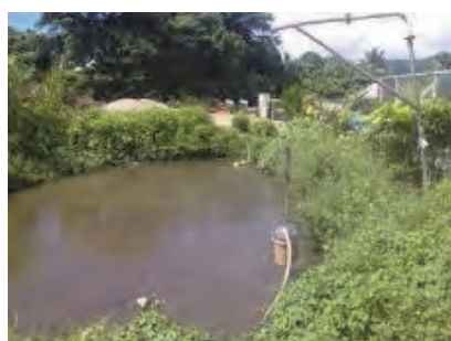
Quality of the leachate has been improved. Color of the leachate has been changed from dark black to green. A leachate recirculation pump was installed.
