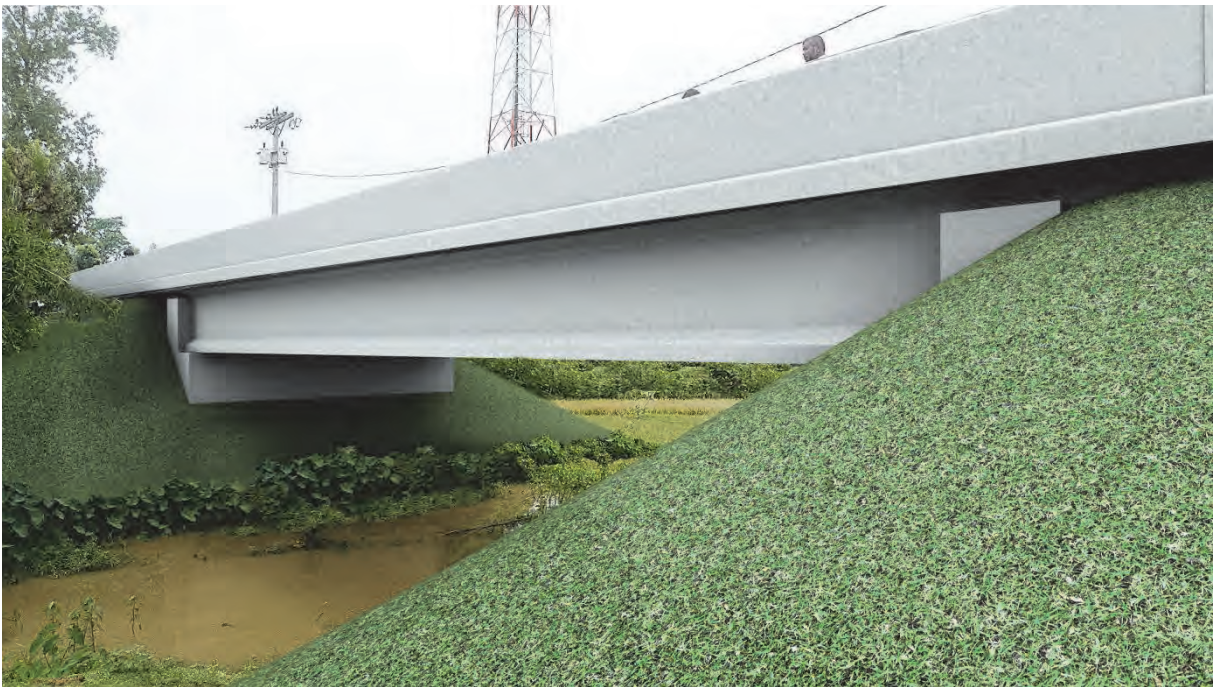
View of PC-I Girder Bridge under Section B
