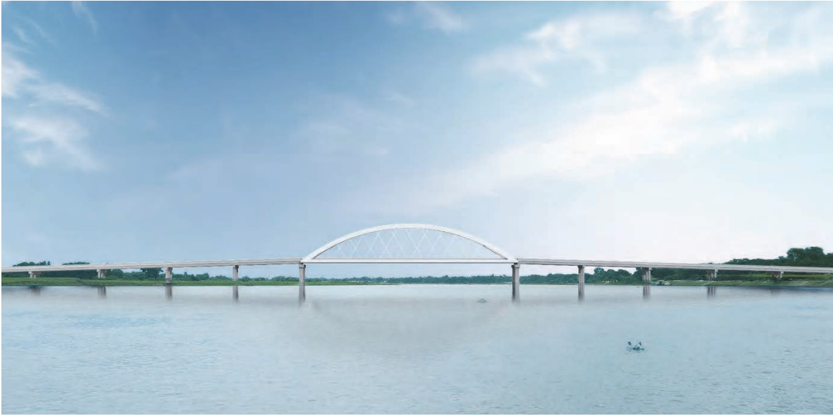
View of Kalna Bridge
