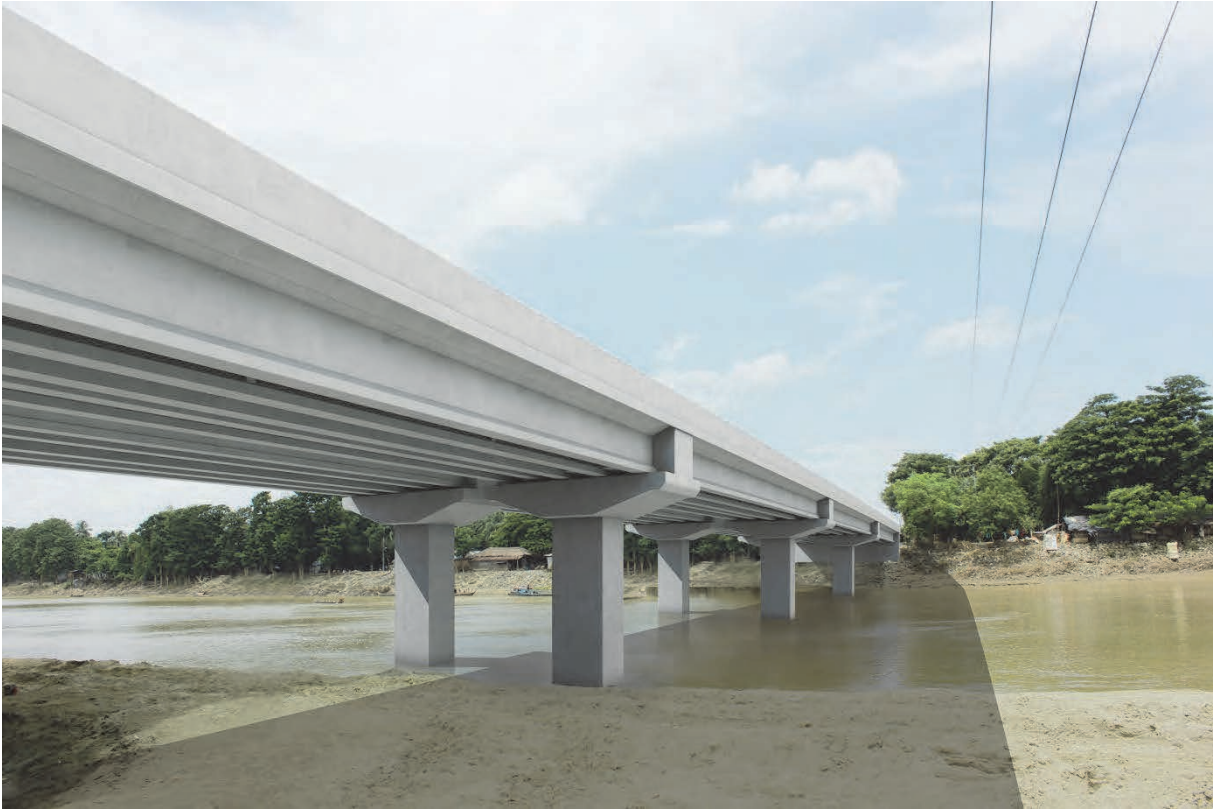
View of PC-I Girder Bridge under Section C
