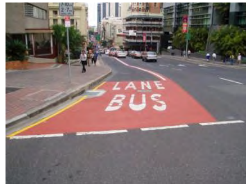
Figure 19. Priority 'jump' lanes also can be used at intersections to prioritise buses in the queue
