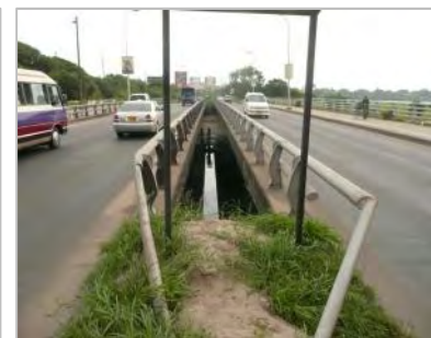
Figure 10. Centre of Bridge
