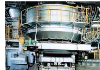
Ash melting facility
