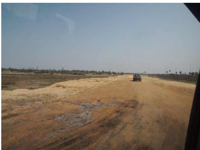
Figure 3.25: Existing Access Road
