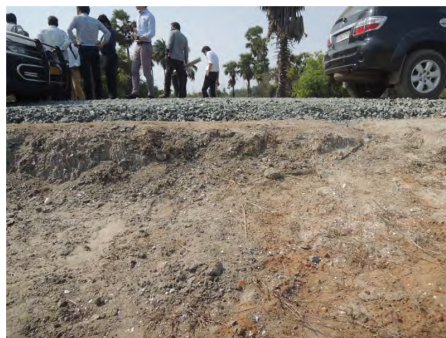
Figure 3.26: : Subbase of the Access Road
