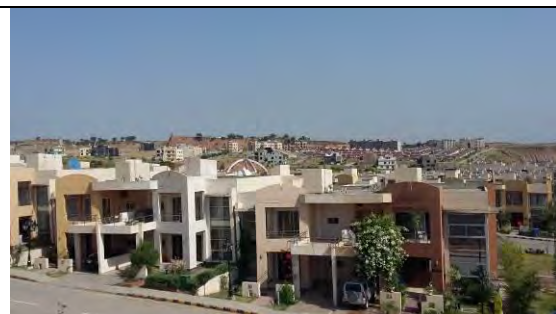
5: New housing scheme in Rawalpindi Typically, 2 storey RC buildings with flat roof
