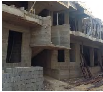
12: Construction in Karachi Concrete block wall is common in Karachi.
