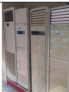
29: Freestanding AC Freestanding AC are often seen in commercial facility where large cooling capacity is required.
