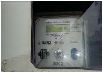
15: Watt hour meter Usually, Consumer can know amount of energy consumption by Watt hour meter
