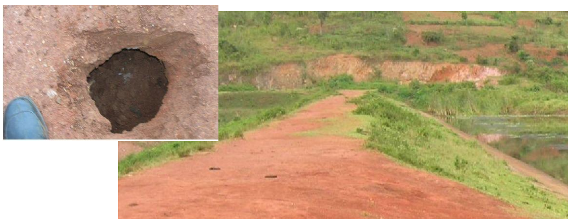
Figure 5.2.4.4 Nests of ants on the dam crest in Rwanda
