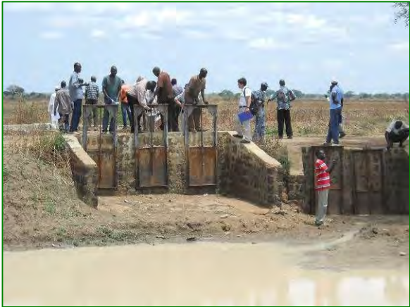
Field Investigation: Aweil Irrigation Rice Scheme
