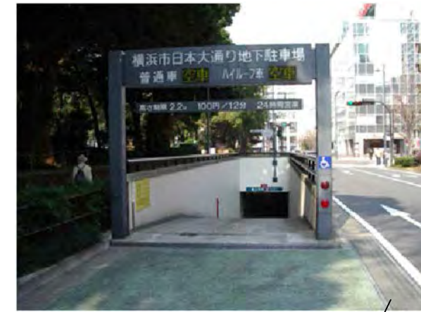
■ UNDERGROUND TRAFFIC ENTRANCE
