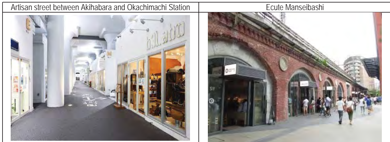
Figure 2.2.18 Examples of Commercial Use under Railway Viaduct
