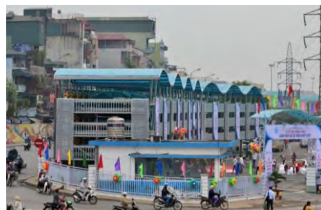
Figure 5.2.1 Multi-Storey Parking on Tran Nhat Duat Street
