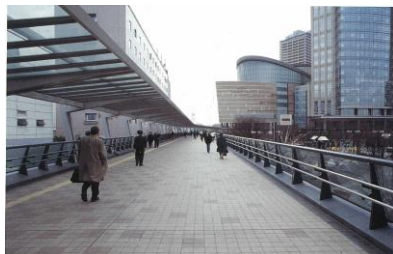
Elevated Walkway Connecting Station and Commercial Area, Kawasaki Skywalk
