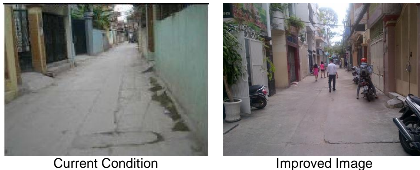
Current Condition Source: JICA Project Team
