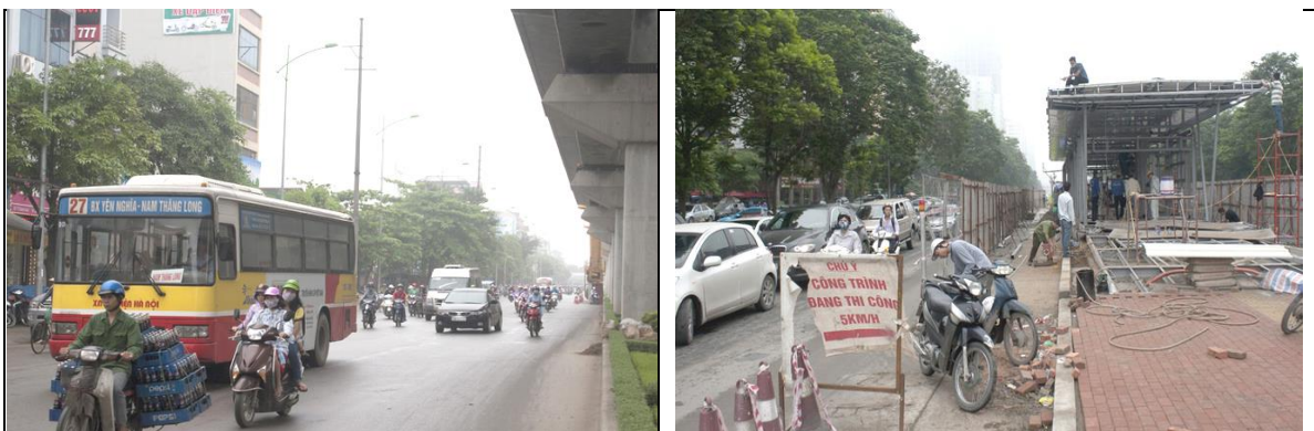
Figure 2.2.23 Roads with Unsegregated Traffic and BRT Shelter Construction
