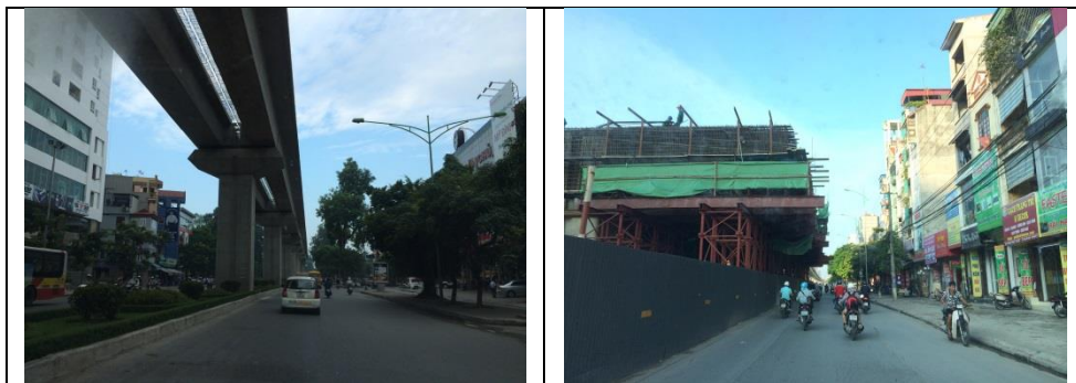
Figure 2.6.2 Photos of UMRT Line 2A Construction Sites
