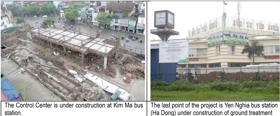
Figure 2.2.21 On-going Construction of Kim Ma and Yen Nghia Bus Stations
