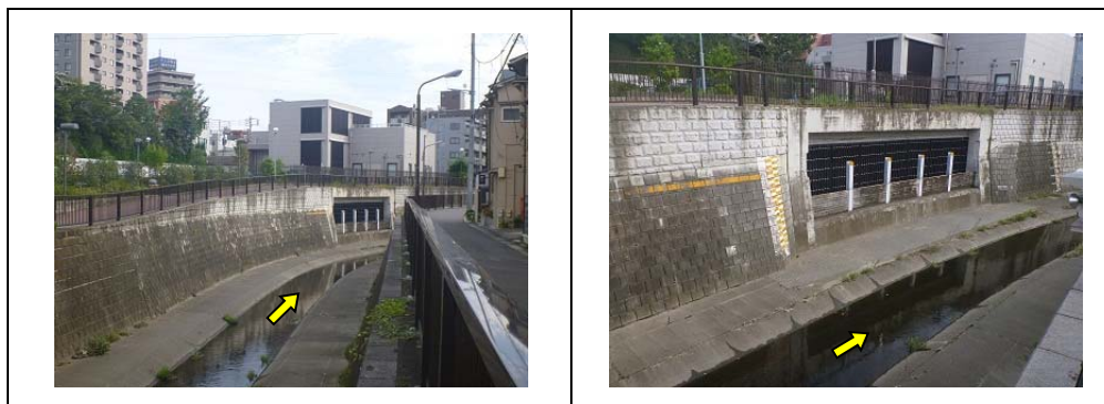
Figure 4.3.14 An Example of Intake Facility (Ring Road No.7 Underground Storage Pipe, Myoshoji-gawa Intake in Tokyo)
