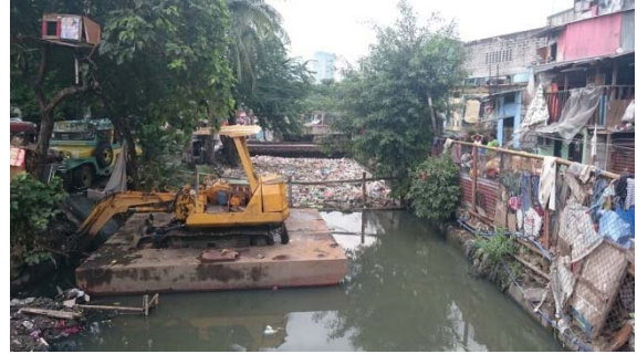
Figure 3.2.12 Dredging in Channel Space
