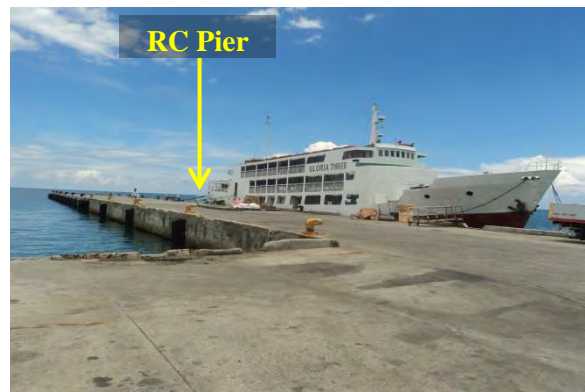
Figure No.7 Existing RC Pier
