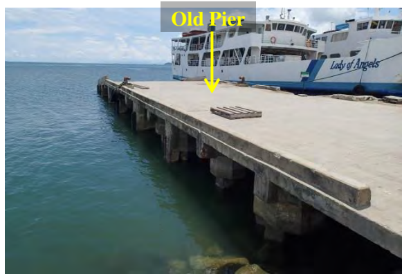
Figure No.2 Left side of the old RC Pier
