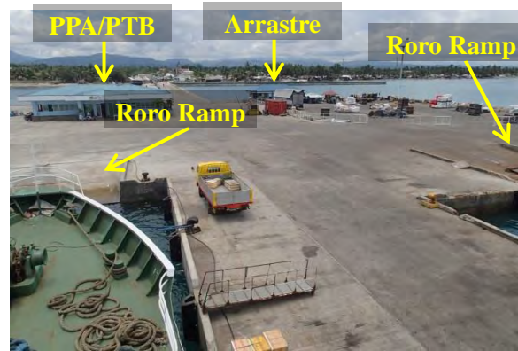
Figure No.3 Port Back-up area at the SE side.
