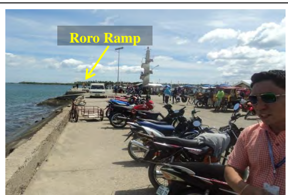
Figure No.3 Damaged causeway pavement caused by OCT 2013 EQ. Causeway is submerged during high tide.
