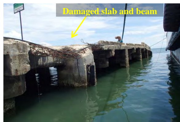
Figure No.3 Right Side of the old RC Pier
