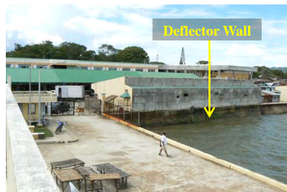
Figure No. 7 Wave Deflector wall.
