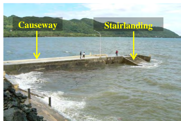
Figure No. 9 Existing Causeway with Stairlanding
