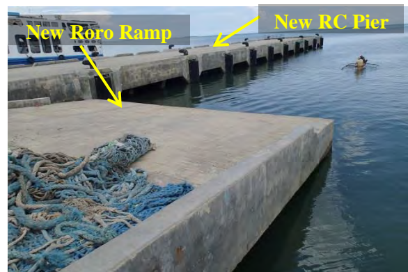
Figure No.7 Right side of the new RC Pier.
