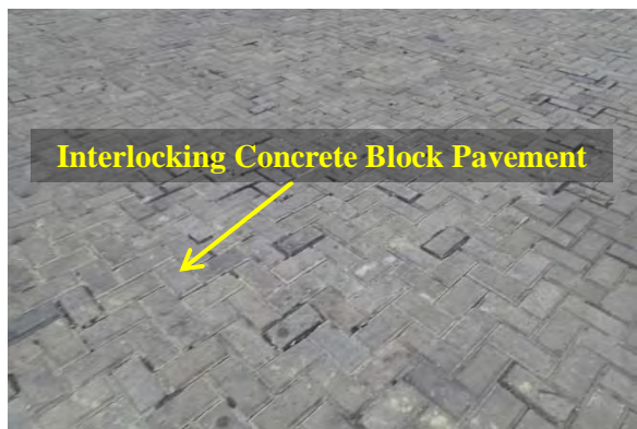
Figure No.10 ILB Pavement used at open storage area.
