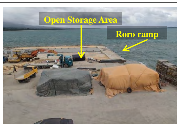
Figure No.3 Open Storage area and the new Roro ramp.
