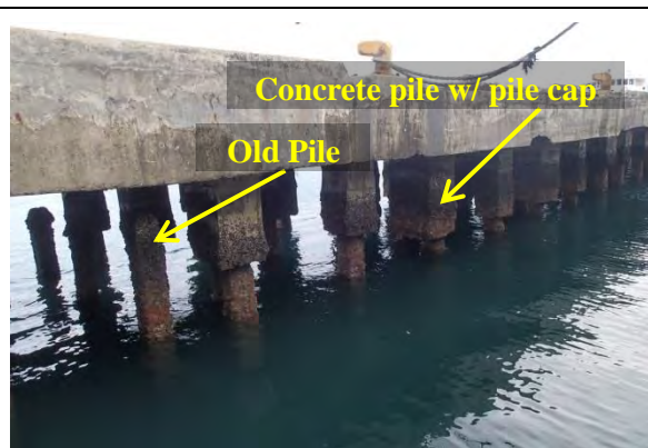
Figure No.3 Right Side of the existing pier.
