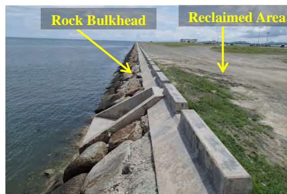
Figure No.11 Rock Bulkhead at reclaimed area
