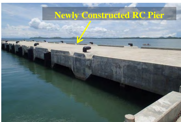
Figure No.6 Left side of the new RC Pier.
