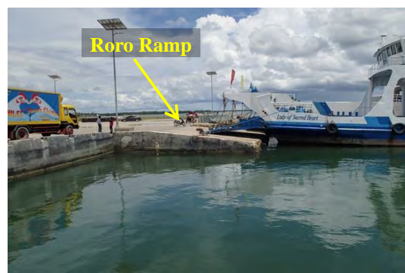
Figure No.5 Roro ramp adjacent to the old RC pier.
