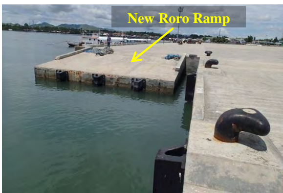
Figure No.8 New Roro ramp.
