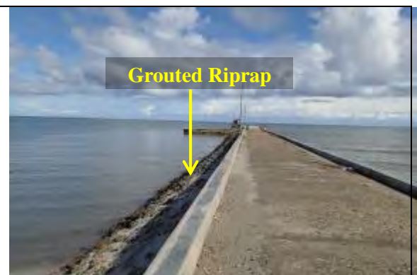
Figure No. 3 Existing Causeway with grouted riprap bulkhead.
