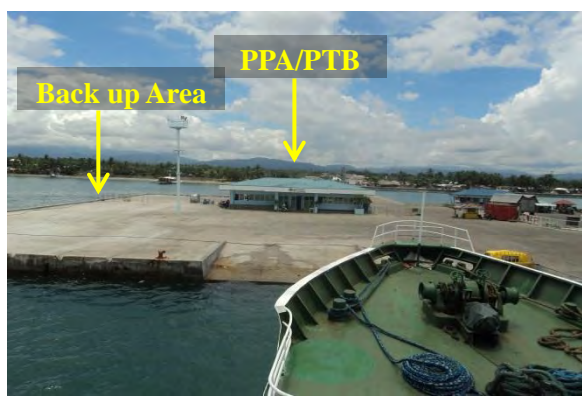
Figure No.2 Port back-up area at the NW side.
