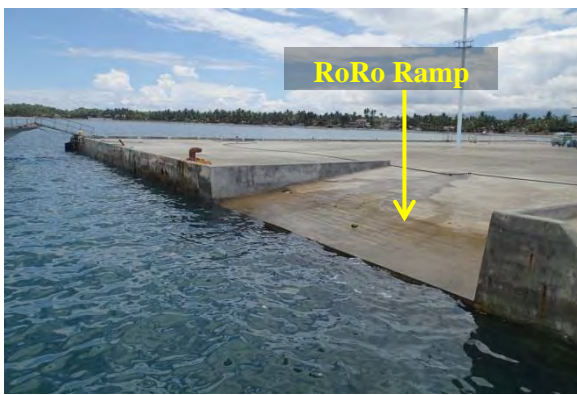
Figure No.4 The RoRo ramp at the west side of the port during high tide.
