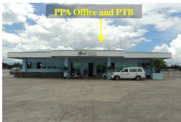
Figure No.12 Photo shows PPA Admin Office and Passenger Terminal Building.
