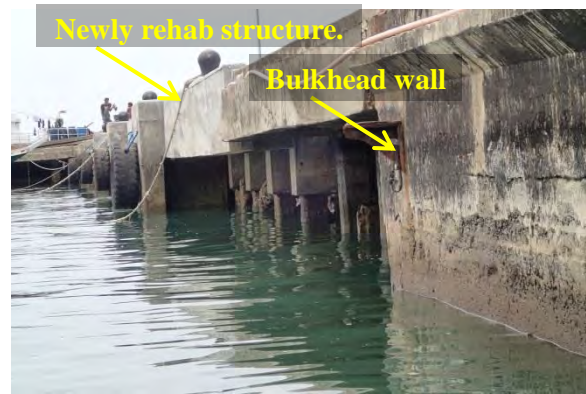
Figure No.5 Figure shows portion of the newly rehab structure.
