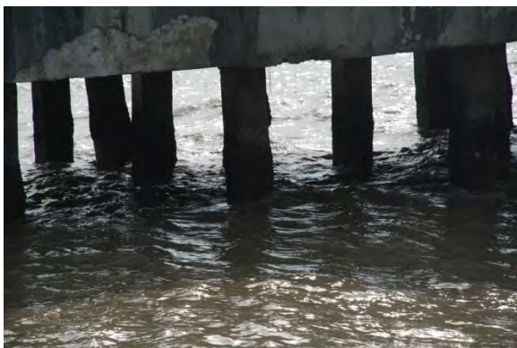
Figure No.6 Condition of RC Piles foundation of RC Trestle.
