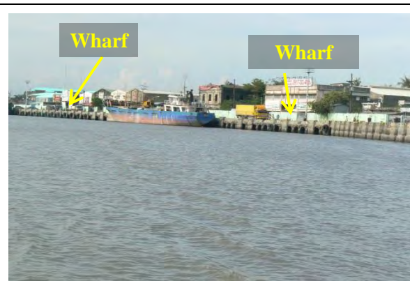
Figure No.3 Existing River Wharf
