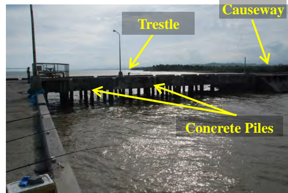
Figure No.5 Existing Causeway and RC Trestle.
