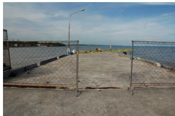
Figure No.7 Existing RC Wharf.
