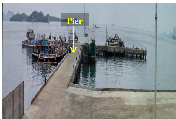
Figure No.2 Access Trestle
