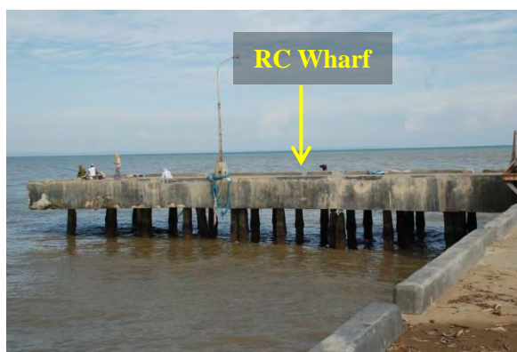
Figure No.2 Existing RC Wharf
