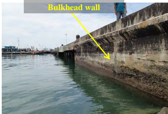
Figure No.4 Bulkhead wall connecting RC Pier/ Trestle.
