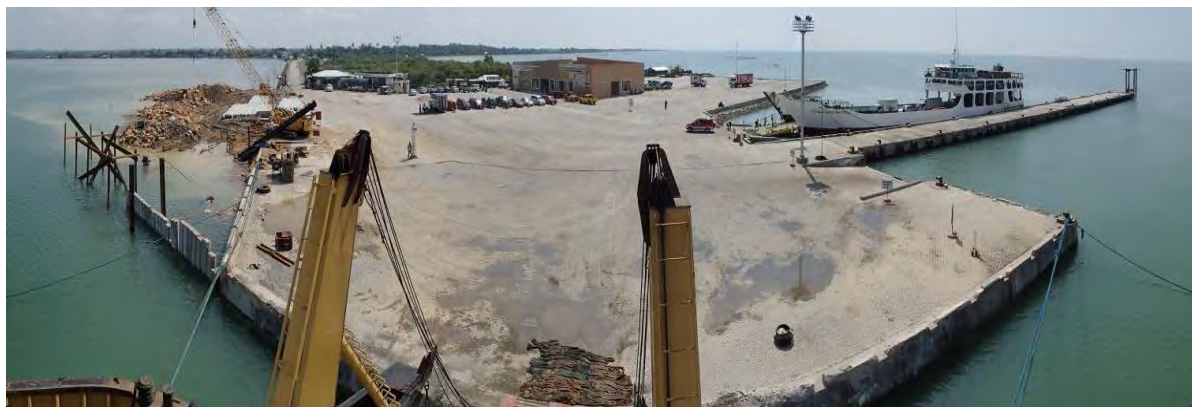
Figure No.2 Panoramic View of Dumangas Port
