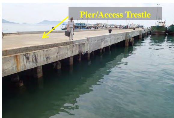
Figure No.6 Newly Rehabilitated Pier/Trestle.
