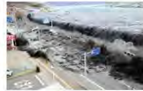
Tsunami overflow the seawall in North Japan
