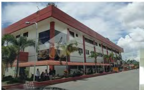
PMO Admin. Office renovated.
