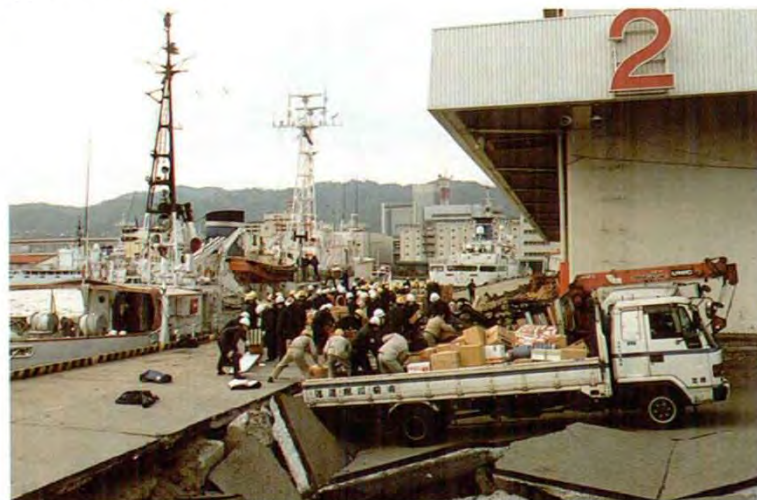
Kobe Port Revival –Overcoming damage from 1995 Southern Hyogo Earthquake/ Kobe City
