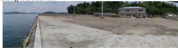
Repaired conc. pavement along the seawall
