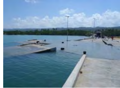
Figure 5.1-6 Damage of liquefaction
