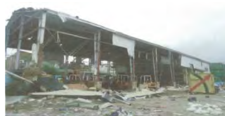
Figure 5.1-4 Damage of Wall by Storm Surge
