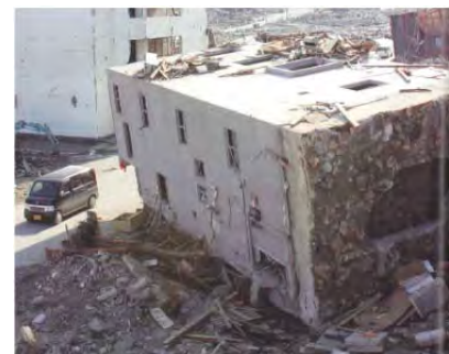
Figure 5.1-8 Damage by Tsunami Pressure
