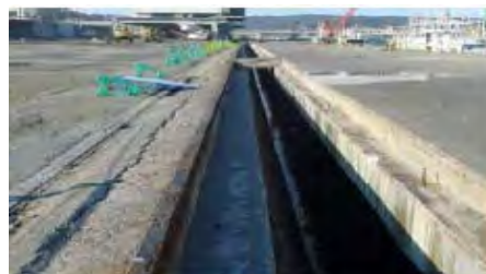
Figure 5.1-3 Damage of Connection Slab by High Wave
