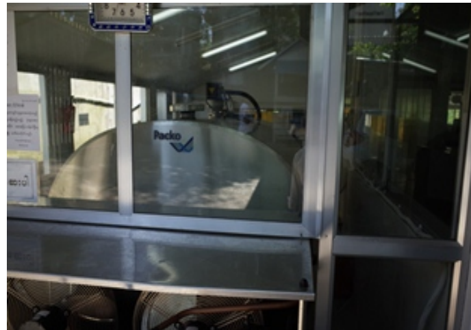
Milk processing facility
