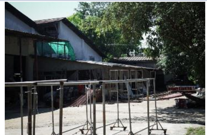
Site for a newly planned factory building 18
