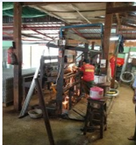
Manual Welding Process
