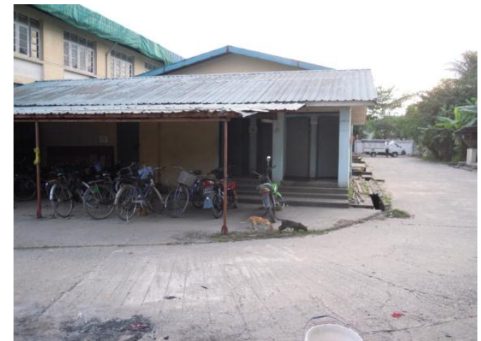
Site for planned factory expansion
