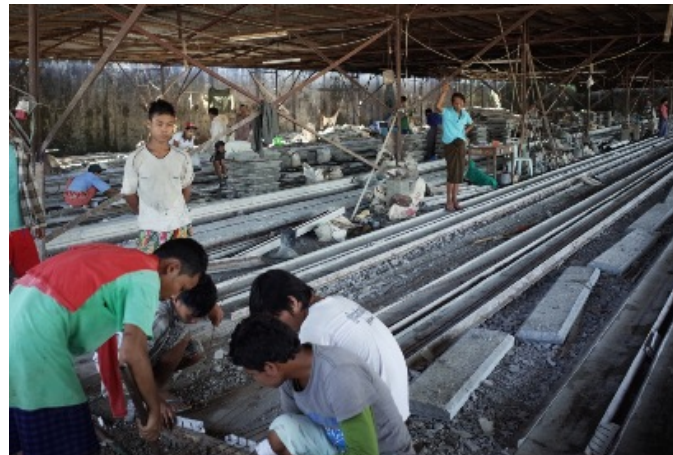
Concrete slab manufacturing site
