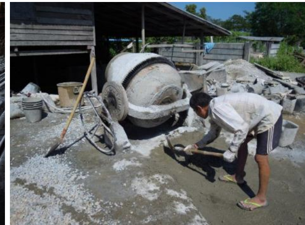
Concrete mixer in current use 2
