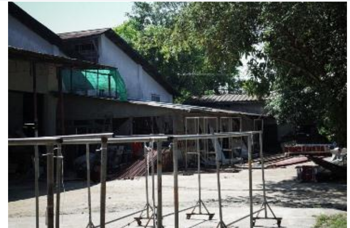
Site for a newly planned factory building 18
