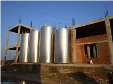
Private milk factory under construction
