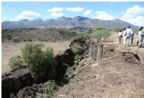
Open crack with a width of more than 10 m at 2 km north of Lake Beseka. L-BA30
