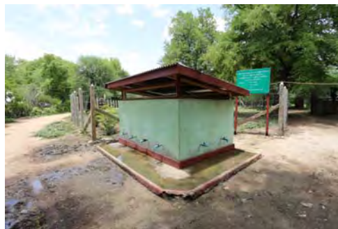
Water Storage Tank
