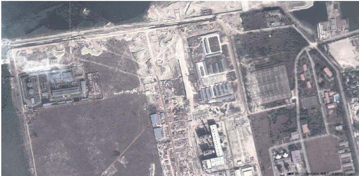
Figure 4.2.1-2 Site Location for Existing 230 kV Meghnaghat Switch Station
