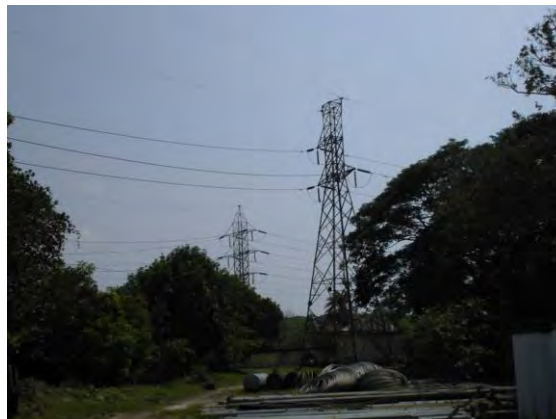
(b) Existing 132kV Hathazari T/L tower on the premises
