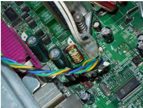
repaired motherboard of HMI terminal
