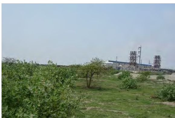
(Source: Taken by the JICA Survey Team)
