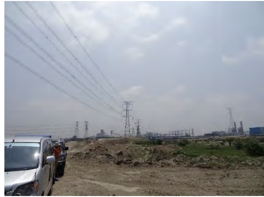
Existing 230 kV Meghnaghat SS
