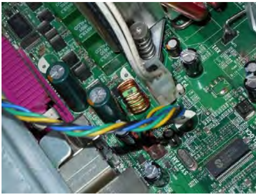
repaired motherboard of HMI terminal
