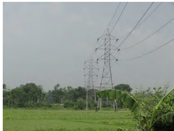
Existing 132 kV Transmission Line
