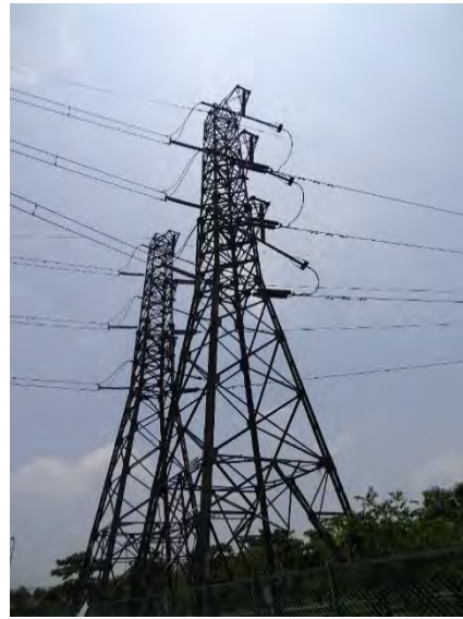
Existing 230 kV T/L Towers (left) River Crossing Tower, (right) Anchor Tower
