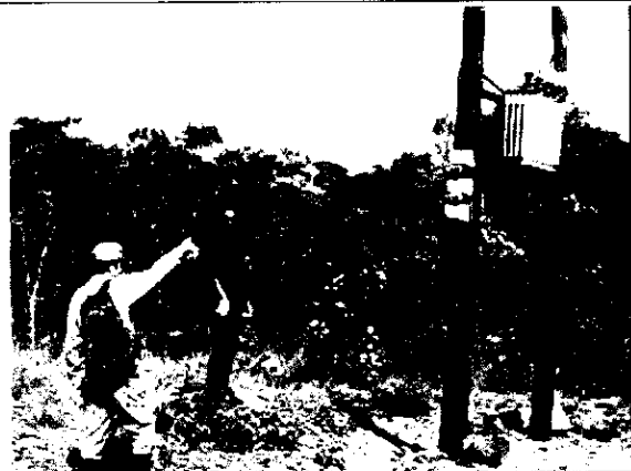
Checking the grid connecting point (Kabompo Dist.)
