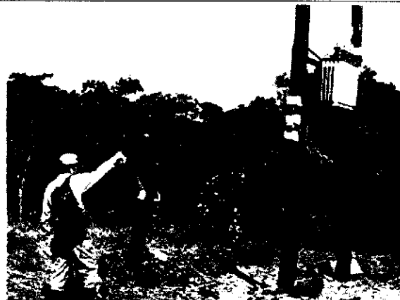
Checking the grid connecting point (Kabompo Dist.)
