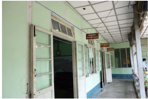
Photo: Corridor of the Entrances
