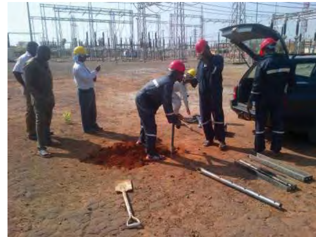
PICTURES OF WORK ON THE PROJECT SITE
