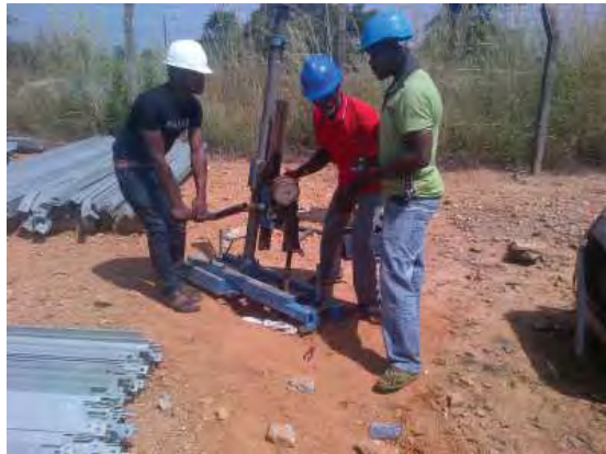
PICTURES SHOWING FIELD OPERATION ON THE PROJECT SITE
