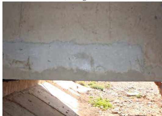
Photo 2.4.47 After Section Repair (ID-41)
