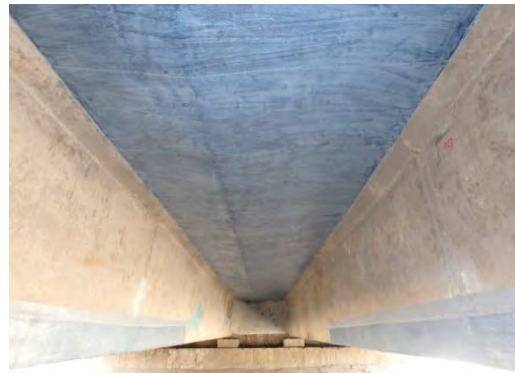
Photo 2.4.49 After Retrofitting on Deck Slab (ID-41)
