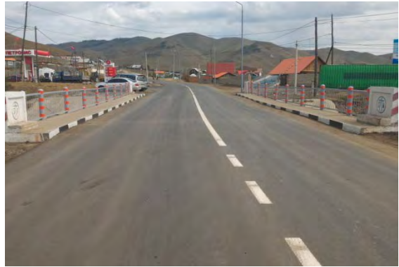
Photo 2.4.45 After Rehabilitation (Bridge Surface: ID-41)
