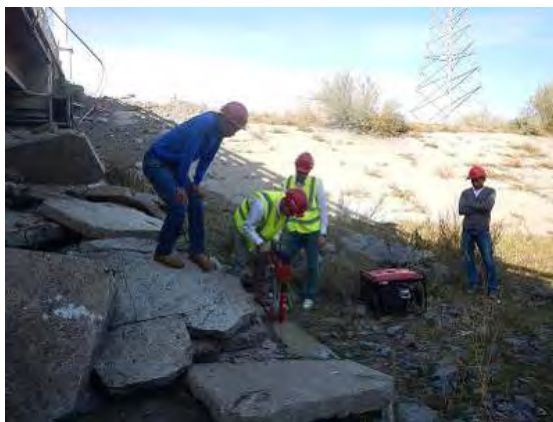
Photo 2.4.5 Training on Core Drilling Machine
