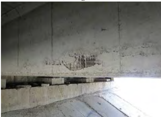
Photo 2.4.46 Before Section Repair (ID-41)
