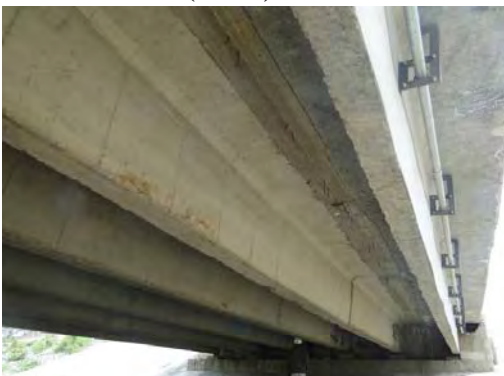
Photo 2.4.50 Before Retrofitting on Main Girder (ID-41)
