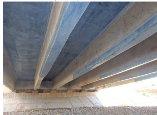
Photo 2.4.51 After Retrofitting on Main Girder (ID-41)
