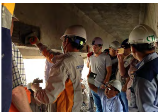
Photo.2.4.42 Technical Assistance in Section Repair
