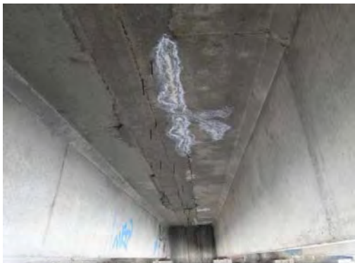
Photo 2.4.48 Before Retrofitting on Deck Slab (ID-41)
