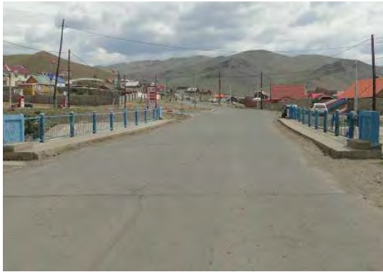
Photo 2.4.44 Before Rehabilitation (Bridge Surface: ID-41)
