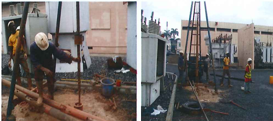
Plate_1: Borehole Drilling In Progress
