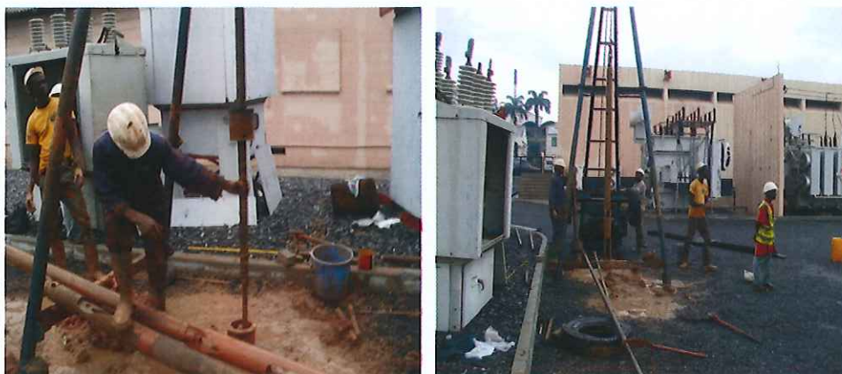
Plate_1: Borehole Drilling In Progress
