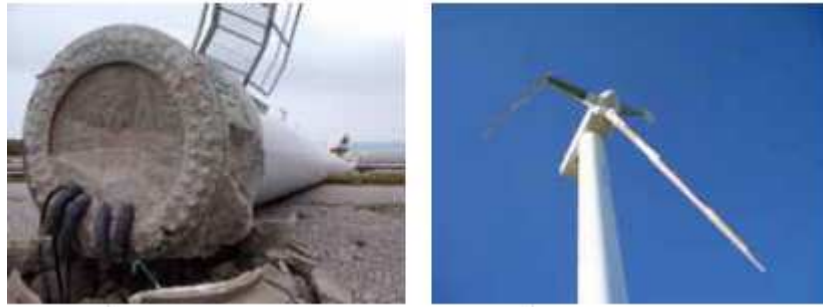
Fig 6-1 Damages to OEPC's Windmills Caused by Typhoon
