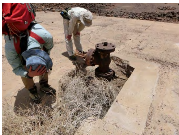
Existing test well in Garabbayis (Garabbayis-2)
