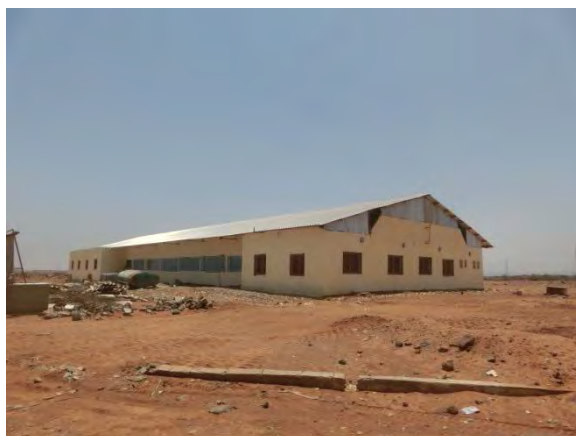
Outside view of ODDEG new head office (under construction)
