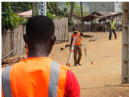
GCP survey (Leveling)
