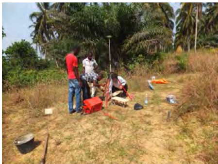
GCP survey (GPS observation and aerial signal)
