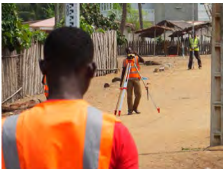
GCP survey (Leveling)
