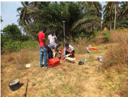
GCP survey (GPS observation and aerial signal)
